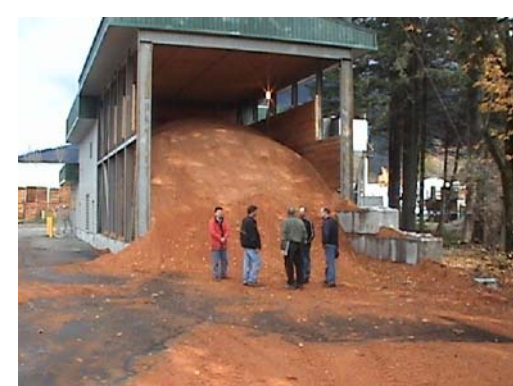
11 RCEC ENERGY CENTRE
